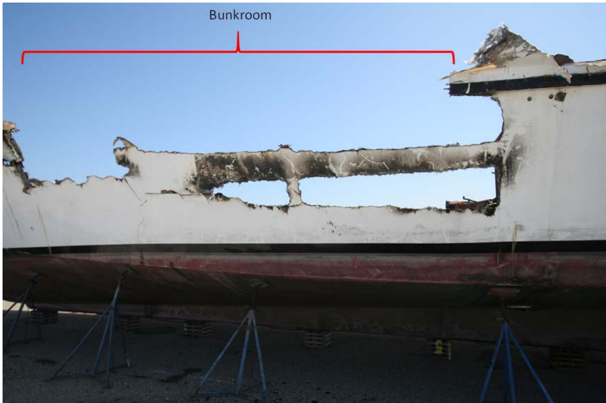
Figure 19. Port-side mid-section of the Conception hull. (Source: FBI ERT)
